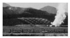
enters perforated pipe and is carried by gravity to open ponds for final extraction of gold and silver.
