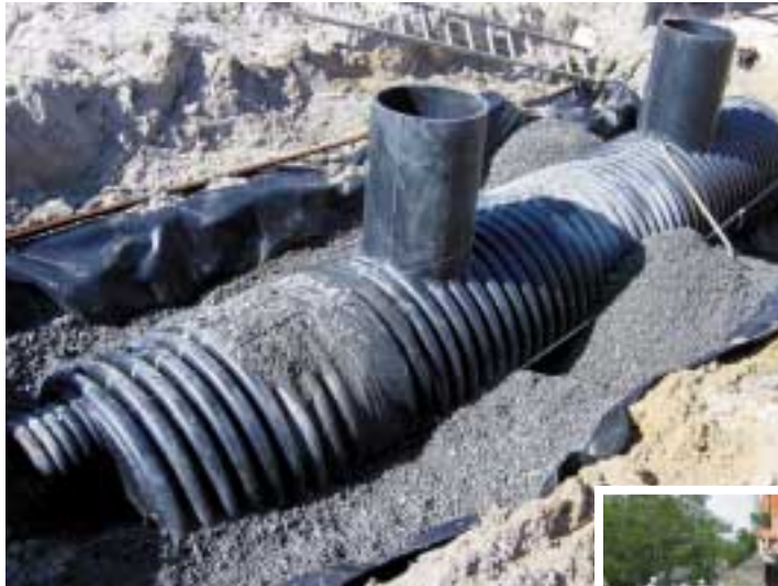
The Patent Pending ADS Water Quality Unit is lightweight and easy to install, requiring little in the way of manpower or heavy equipment.
