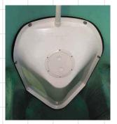
**Design Tip:** To increase water quality benefit, use a larger structure size for a smaller pipe, or increase the sump depth. A bigger deeper structure means more volume for settling and less frequent maintenance.
