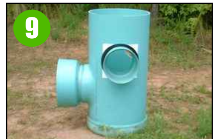
9 Add-a-Branch installation is complete and ready for pipe to be inserted.
