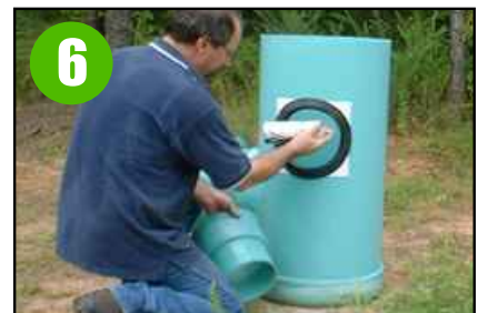
6 Once the Add-a-Branch gasket is installed, lubricate inner surface with standard pipe lubricant.
