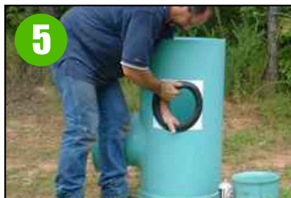
5 Install Add-a-Branch gasket into cut-out hole starting from the bottom and working it around until the inside flange is fit properly.
