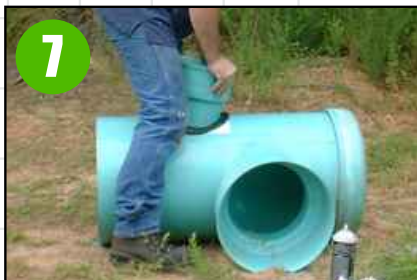
7 Install Add-a-Branch adapter by inserting one edge and twisting while pressing firmly toward the center of the drain basin.
