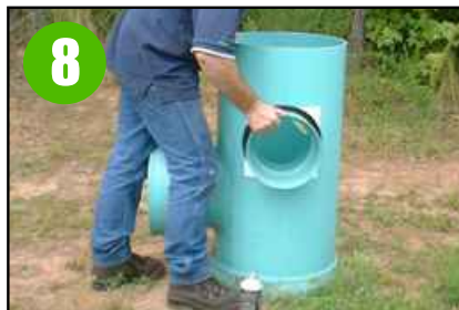
8 Check to make sure it is fully seated into the gasket and straight.
