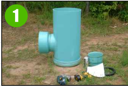
1 Nyloplast Drain Basin ready for Add-a-Branch Installation.
