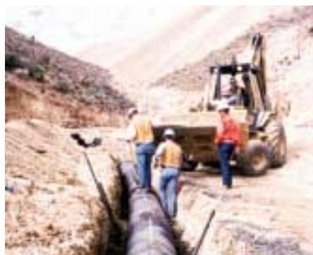
The consulting engineer, Dames and Moore (now URS), believed that corrugated HDPE pipe could handle the acid and abrasion, but were not sure how the pipe would perform at surcharge pressures of 833 psi under 1,000 feet (300m) of crushed ore.
